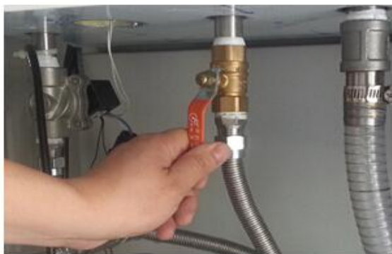
Turn on the drain valve, and discharge all water of working room.
